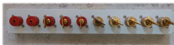
Figure 3: Mechanical "Castell" trapped key exchange interlock.
