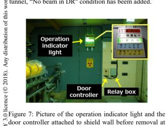
Figure 7: Picture of the operation indicator light and the door controller attached to shield wall before removal at the dividing point of Linac.
