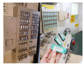
Figure 5: Picture of integrated personal key box (left), downstream personal key box (top right) and a personal key (down right).
