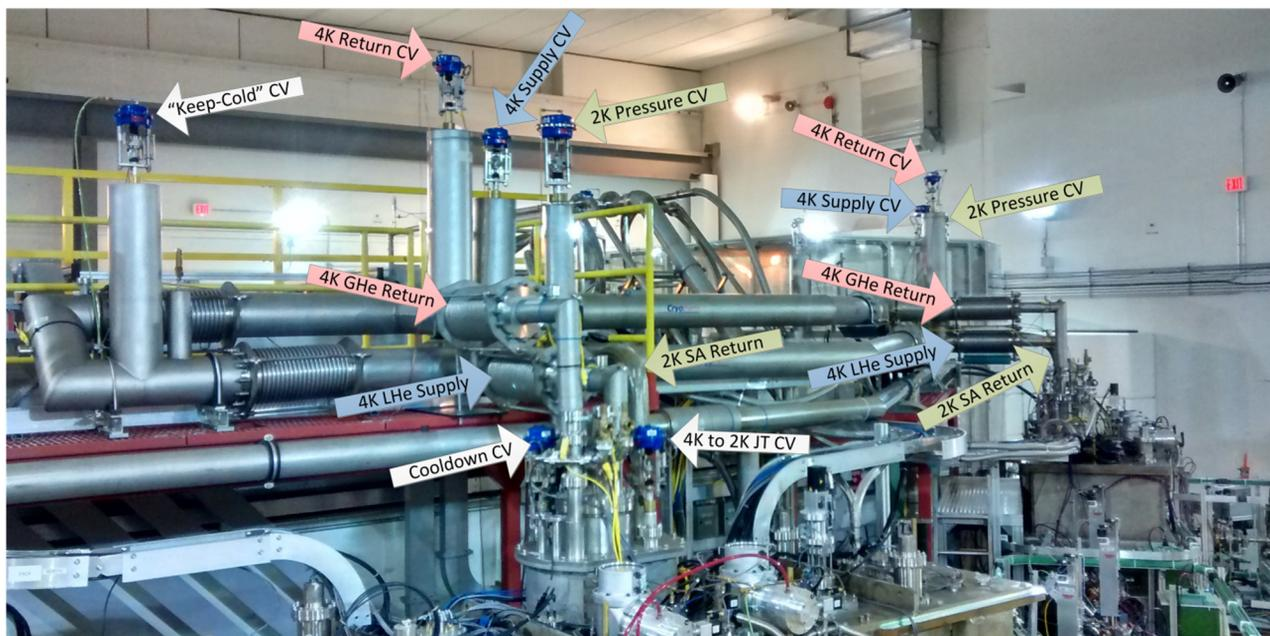
Figure 2: Close-up look at the modular liquid helium distribution system and sub-atmospheric return system around accelerator cryomodule (indicated cryogenic valves).
