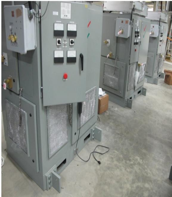
Figure 3: TPS quadruple magnet power converters.
