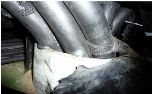
Figure 3: Damaged cable at the vertical shaft, which caused the ground fault.
