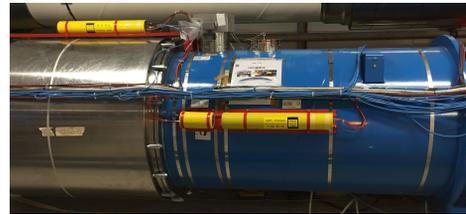
Figure 1: Ionization chamber BLMs installed outside of a LHC dipole magnet.
