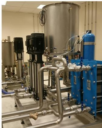
Figure 8: The cooling system installed for the METU-DBL in the technical room. The cooling system has a tank, heat exchangers and pumps.
