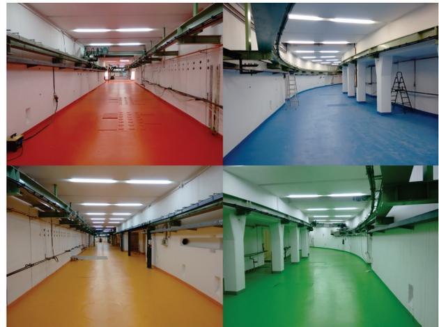
Figure 2: Photos of the current status of the SINBAD accelerator tunnel. The old Doris accelerator and its infrastructure is removed, the building structure refurbished and the installation of the new infrastructure has started.
