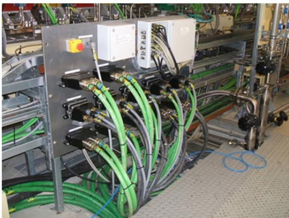
Figure 3: DDBA girder connector panels.
