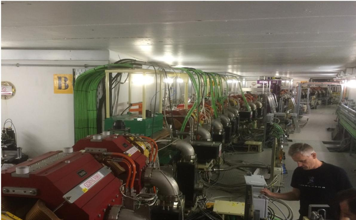
Figure 2: Temporary cables connected to existing DBA cell.
