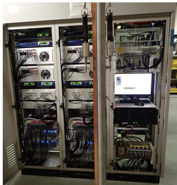
Figure 3: A photo of the standard unit for 4 quadrupole and 4 steering magnets.
