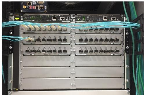
Figure 1: Core switch Aruba 5412R.
