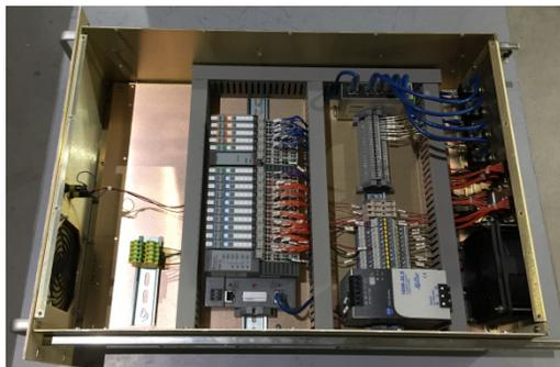
Figure 2: Vacuum interlock chassis module layout.
