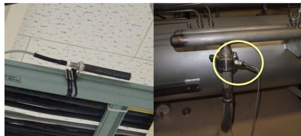
Figure 1: Pictures of the temperature sensor in the klystron gallery (left) and for the cooling water of accelerating structure (right).
