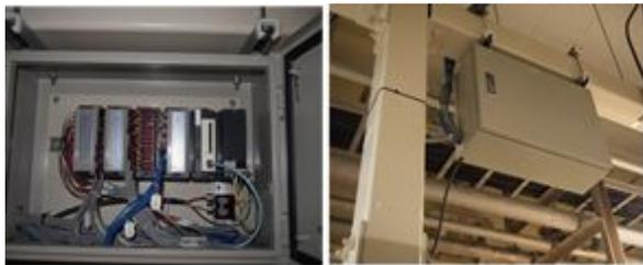
Figure 2: Picture of the data logger provided with the communication unit, power supply unit and input units.
