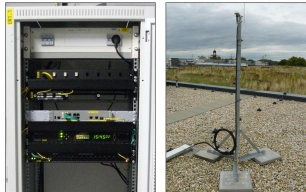
Figure 10: A White Rabbit “Grandmaster” switch is connected to an antenna under their roof.
