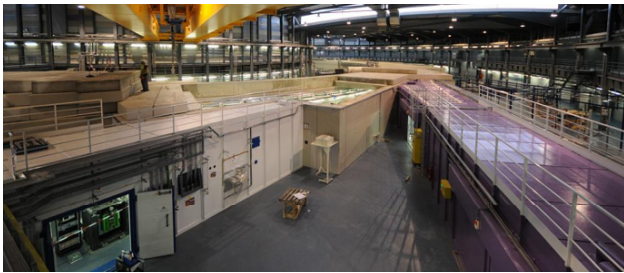
Figure 1: View of the Accelerator tunnel and BL11 and BL13 Beamline hutches. Picture taken on 8 September 2009 (J.Klora).
