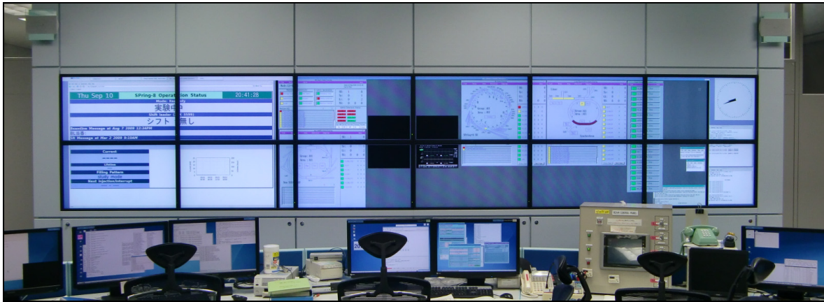
Figure 6: Display wall (SPring-8 Central Control Room). In the center of the display, sub-screens display real-time NTSC video.
