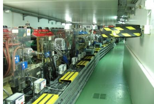
Figure 2: inside the tunnel.
