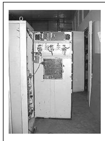
Fig.2: View of the interface card inside the power supply
