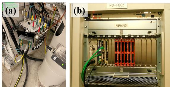
Figure 3: BPM readout system installation in PETRA III: (a) *Libera XBS FE* crossbar switch matrix installation in the tunnel and patch panel for signal splitting; (b) MTCA crate in the electronics cabinet equipped with 6 AMC boards, MCH, CPU, timing and fan module.
