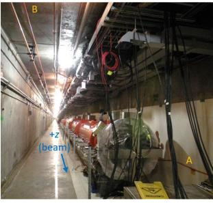
Figure 2: Photo during installation showing the A fibre on the right (north) wall and the B fibre on the ceiling at left. Both are in 6-mm orange "fibre ducts" that allow fibre replacement in a few minutes, without entering the tunnel.
