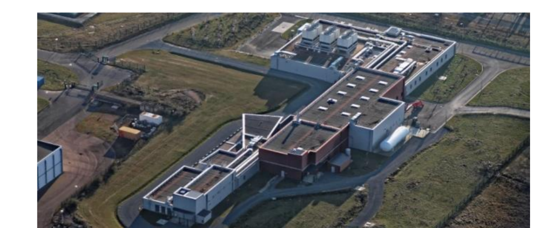
Completion of the SPIRAL2 building (October 2014).
