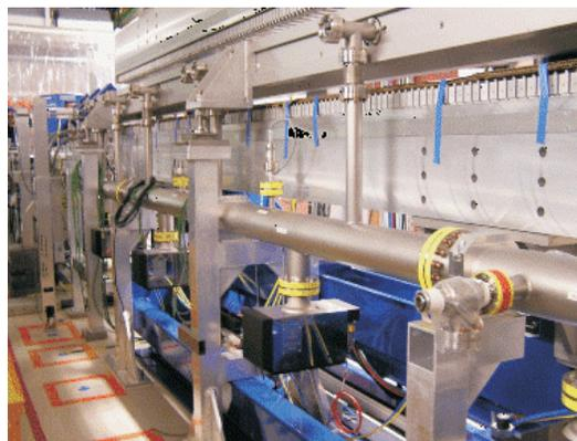
Figure 10: Collective vacuum line with getter pumps and connectors to the waveguide.
