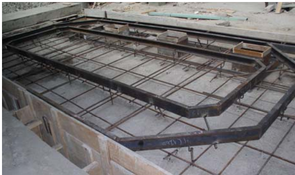
Figure 2: General view of the NESTOR ring foundation.
