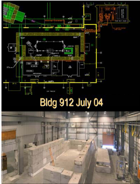
Fig.3 The layout of the facility (top) and the photograph of the shielded vault for R&D ERL under construction in the bay of Bldg. 912. The bay is equipped with an overhead crane. The control room is located outside of the bay in a separate building.
