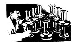
Figure 2. single cell 1300 MHz TESLA type Nb cavities
