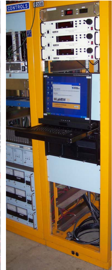
E0 service building
