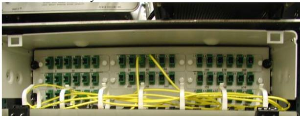
Figure 4: Fiber optic delay box. Users use a fiber to connect specific lengths of fiber.
