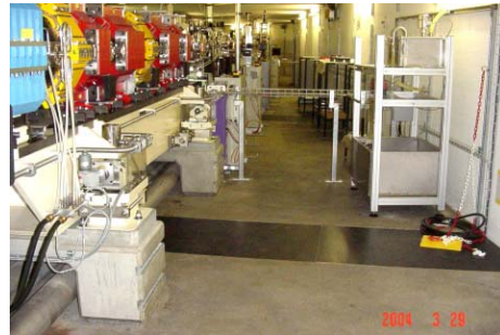
Figure 2: HLS and its filling station.
