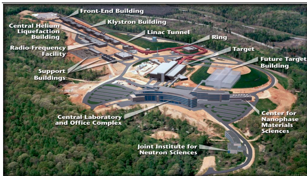
Figure 1: Overview of the construction site with accelerator systems, target buildings, the central laboratory office, JINS, CNMS and several support buildings overlaid on a early site photo on top of Chestnut Ridge at Oak Ridge National Laboratory.
