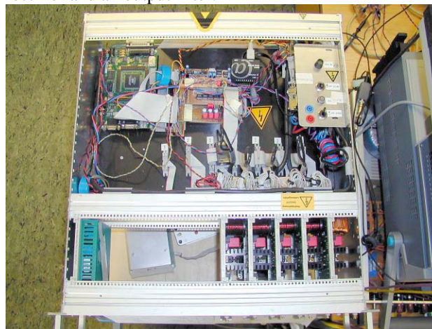
Figure 2: 100A, \pm 10V test rack
