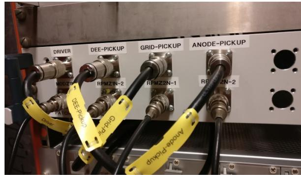
Figure 3: Patch panel for RF signals.
