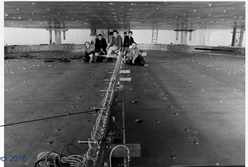
Field mapping using flip coils
