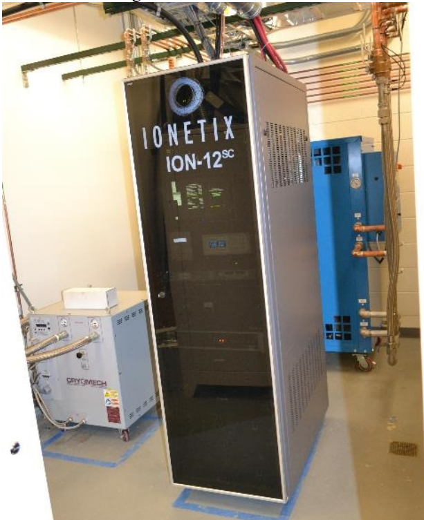
Figure 8: Electronics rack installed at the University of Michigan Medical School.
