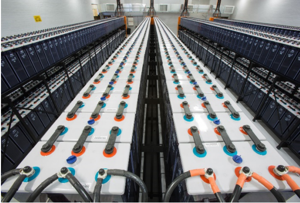
Figure 1: The new 4.4-MVA battery installation.
