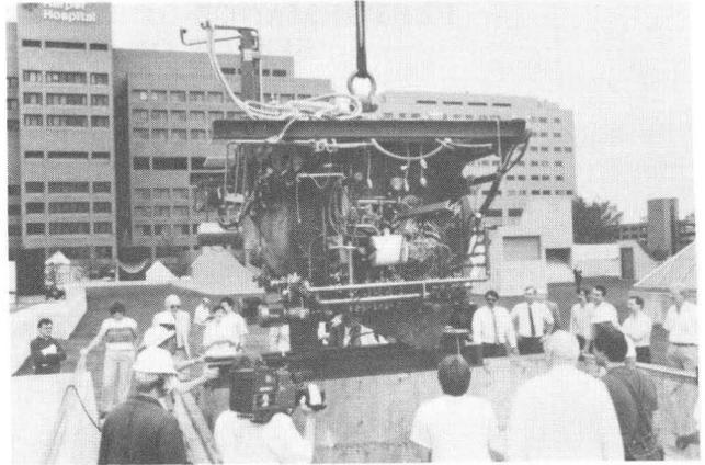
Figure 3. View of the K100 cyclotron being lowered through the roof of the Harper Hospital Oncology Center.
