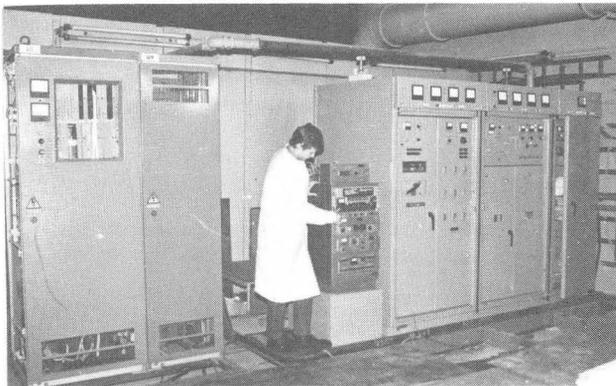
Fig. 3. Magnet main coil power supply (on the left) and RF oscillator (on the right).
