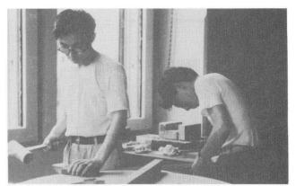
Fig.18 Coil winding works for the proto-type machine. At the left is S.Suwa who was later the 1st director of KEK.
