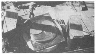
Fig.24 The magnet of the INS-SF cyclotron with the bottom plate of vacuum chamber, removed the top yoke.
