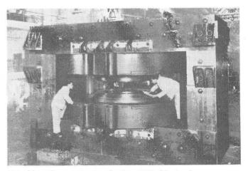
Fig.20 The magnet of the INS 63 inch cyclotron, before mounting the vacuum chamber, 1956.
