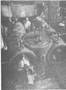
Fig.5 The improved rf resonator and vacuum pump for the 60 inch evelotron. In the left foreground is seen the insulator for deflector high voltage. In the center is Y.Nishina standing.
