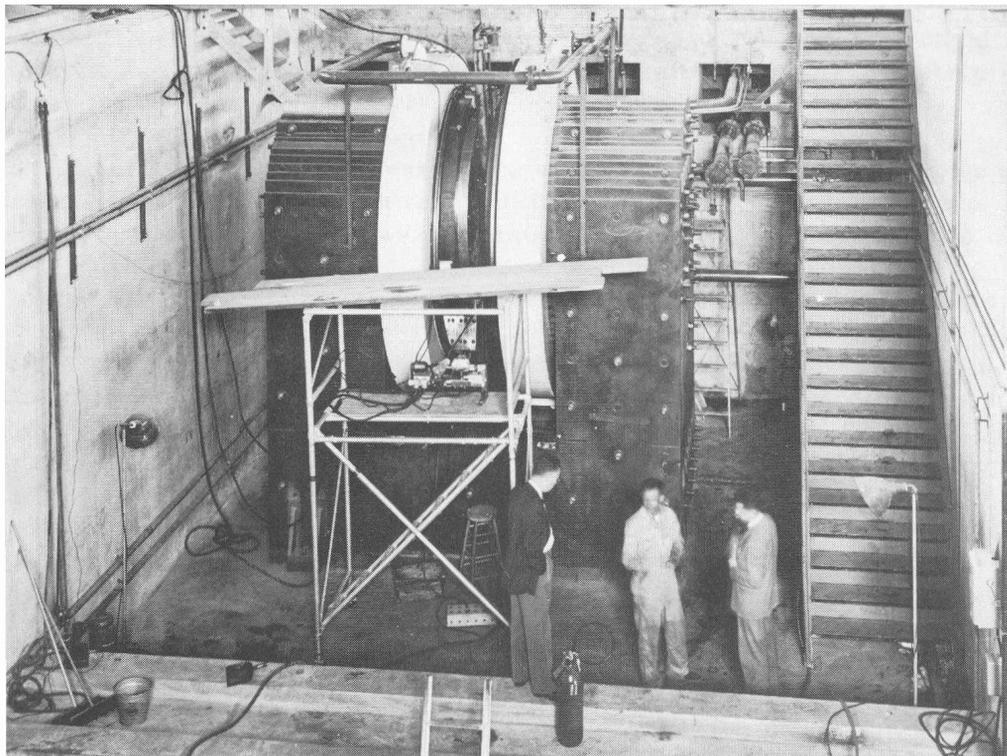
Fig. 201. Livermore cyclotron magnet, shown during construction pole tips and magnet coils in place.
