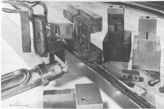
Fig. 177. Ion source hoods and beam defining slits on first three turns.
