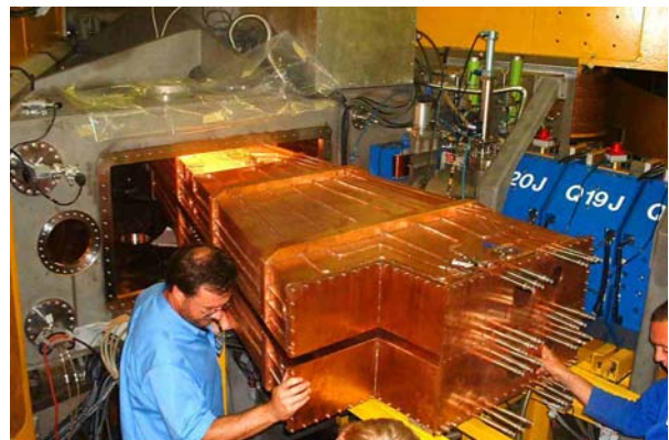
Figure 2: The flattop resonator during installation through a port in the south valley vacuum chamber of the cyclotron. The last two quadrupole magnets of the transfer beam line are visible on the right.
