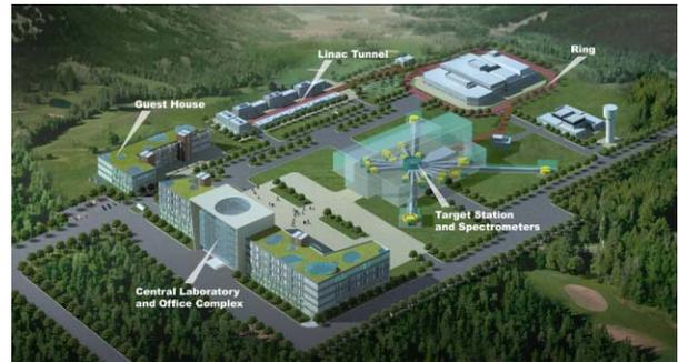
Figure 2: Schematic layout of the CSNS complex (courtesy Institute of Physics, CAS).
