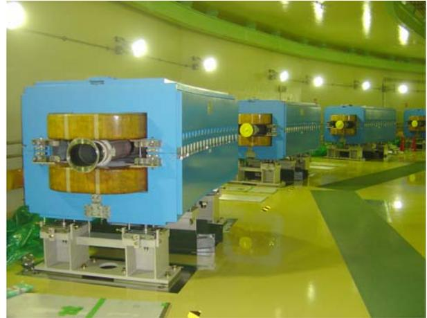
Figure 3: The bending magnets installed to the J-PARC RCS tunnel
