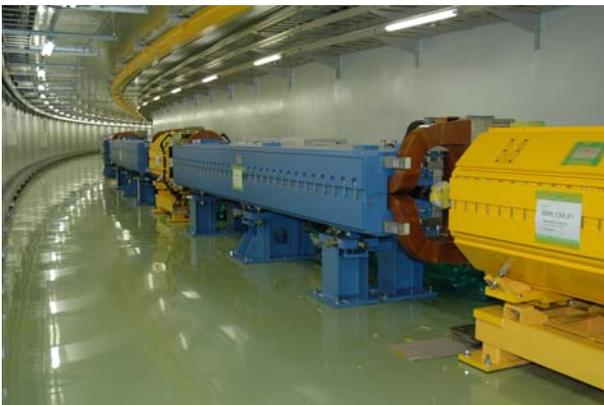
Figure 10: Typical Arc Section in the MR tunnel
