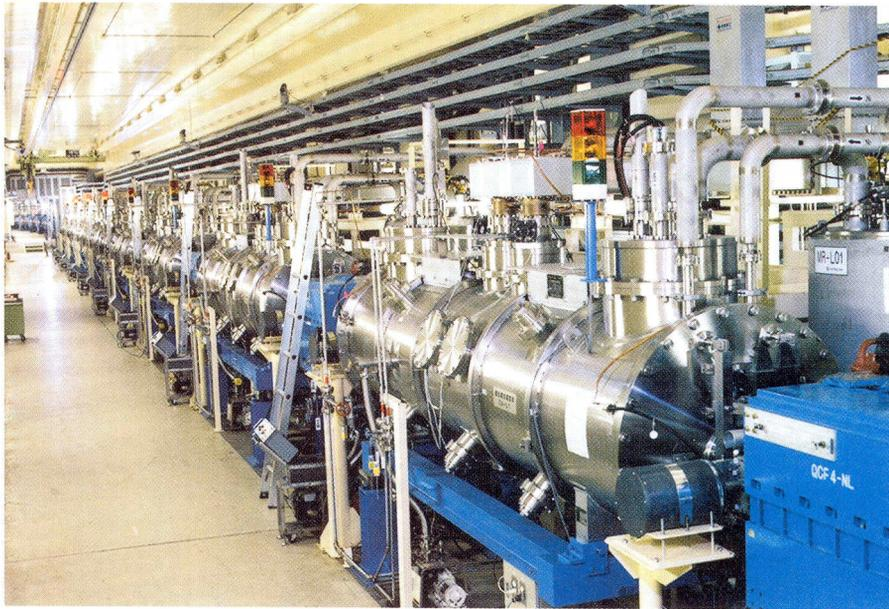
Fig.2 The string of SC cavities in the TRISTAN tunnel
