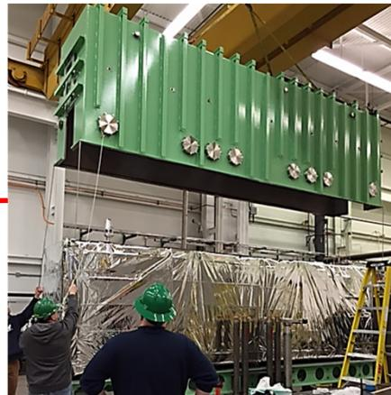
Vacuum Vessel Lift onto Baseplate
