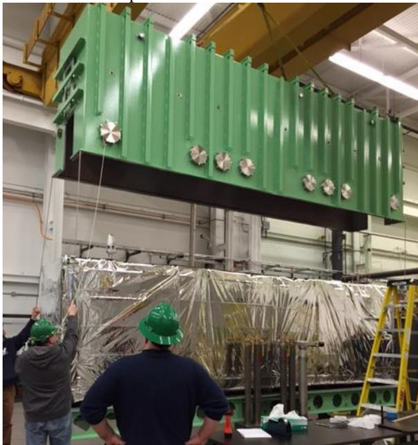
Figure 12: Lowering the vacuum vessel cover into place on the ReA6 cryomodule.
