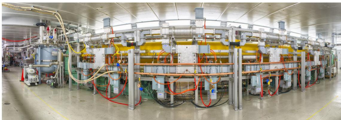
Figure 10: CM-2 installed in the FAST cave at Fermilab. In the foreground is the waveguide distribution system which delivers RF output from a single 5 MW klystron to the coupler of each cavity.
