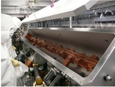
Figure 5: ReA RFQ during the final installation.
