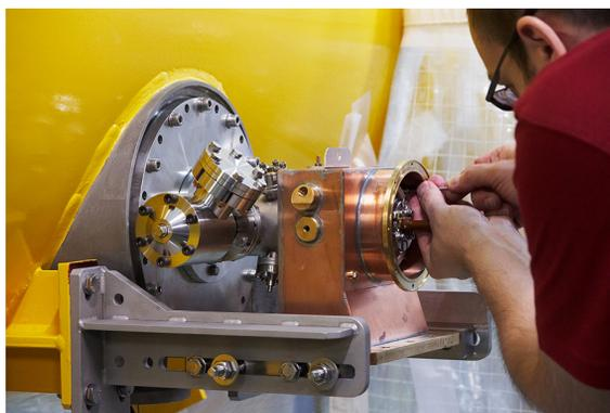
Figure 5: Assembly work of the cryomodules in progress.
