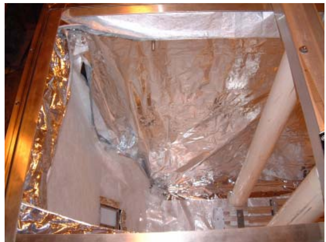
Figure 5: Multi-layer insulation blanket installed between vacuum vessel and thermal shield.
