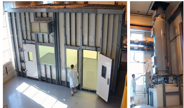
Figure 2: A pair of large chemical processing rooms (left) and an exhaust fume scrubber (right). These facilities are sized to chemically process several cavities per week.
